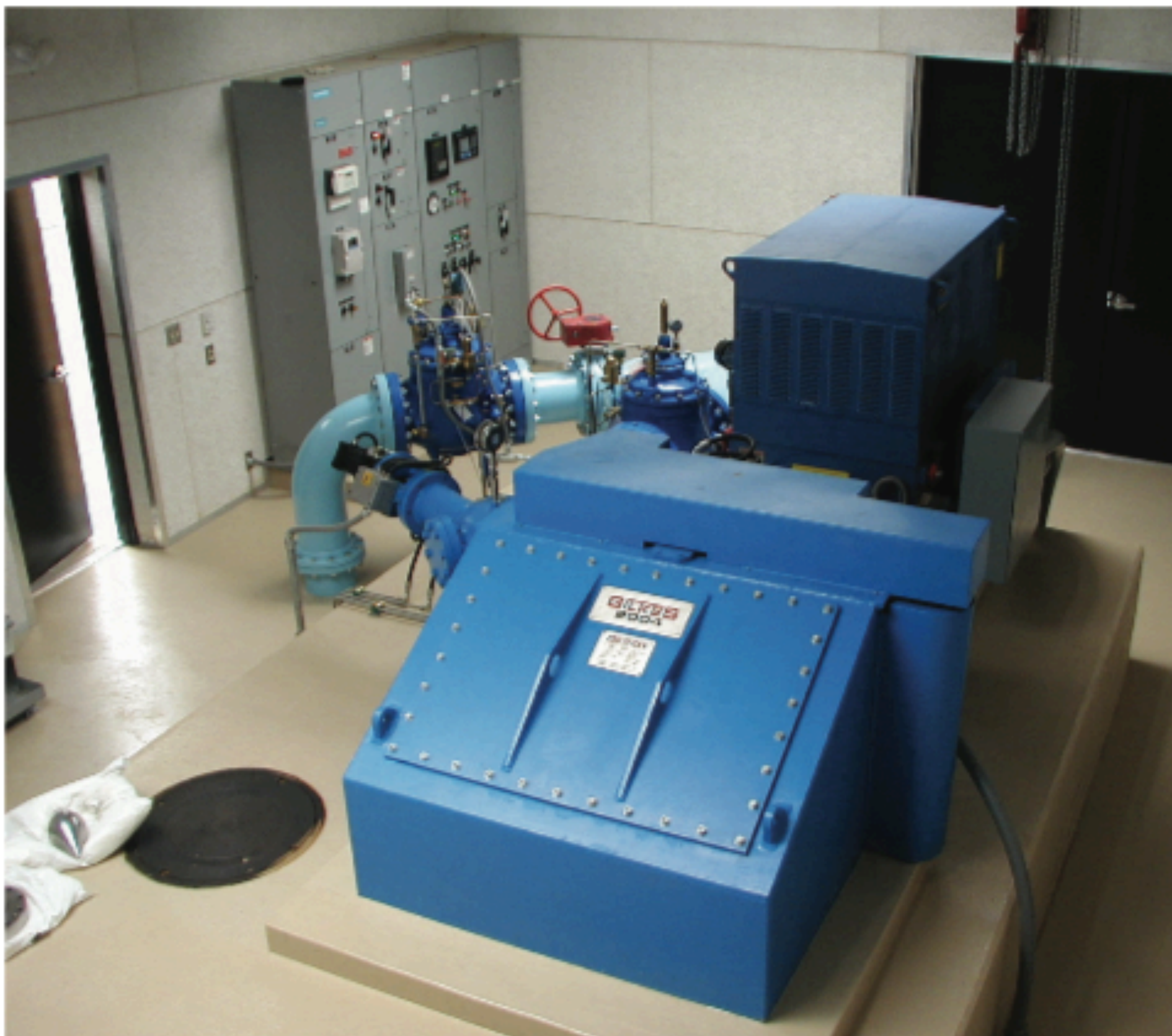
12 Inch mean diameter singlet jet Gilkes Turgo installed at Draper Irrigation Company, UT, USA. Net Head 633ft, Rated Flow 11.7cfs, Speed 1800rpm, Power 511kW, Year 2004
